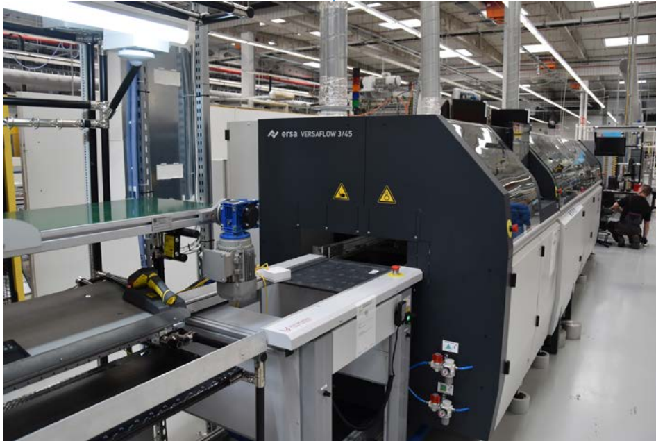
Ersa VERSAFLOW 3/45 at the Jabil production facility in Kwidzyn
